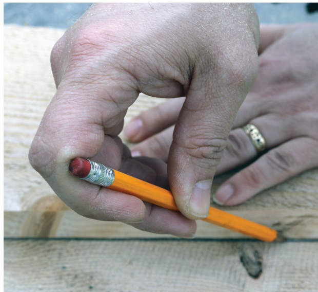
Measure three times, cut once. Note straightedge.
